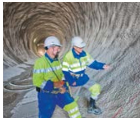
Chemical solutions for underground construction
