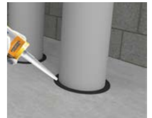
Fire protection systems
